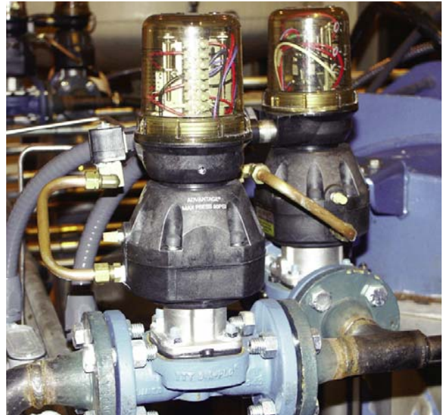
Dia-Flo® weir diaphragm valve with Advantage Actuator and SP2.0 switch pack.
